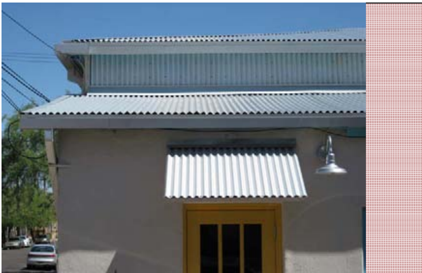
Appropriate: Pitched Corrugated metal roofs of varying height (shown on a Territorial Style building)
