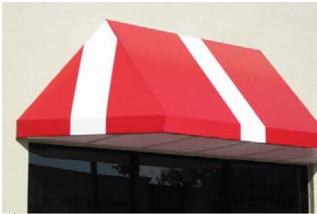
Unfavorable: Awning as a dominant feature that does not complement building
