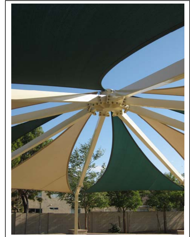
Below: Interior of Multi-panel Hexagon Structure
